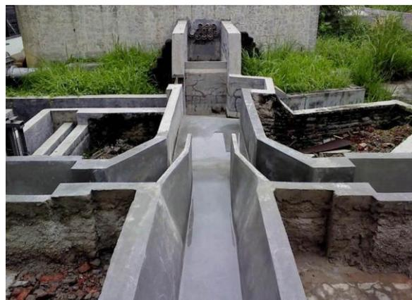
**Gambar 4** Model Fisik Bangunan Bagi Proporsional (Subari et al., 2013)
